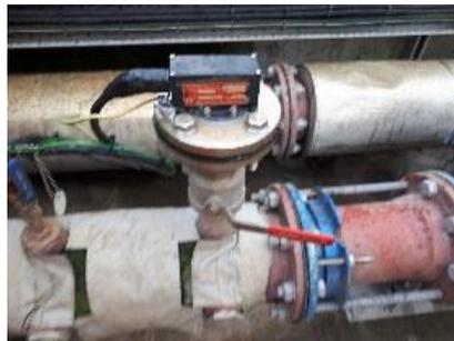
Pressure sensor with isolation valve below
